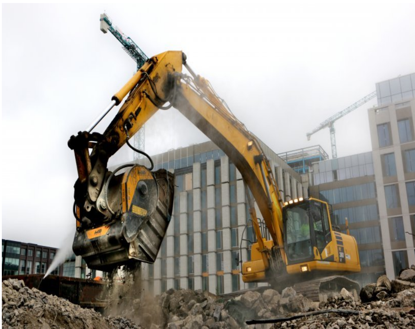
BF120.4 & Komatsu PC360 LC - Ireland, Dublin Port - Recycling - Reinforced concrete
