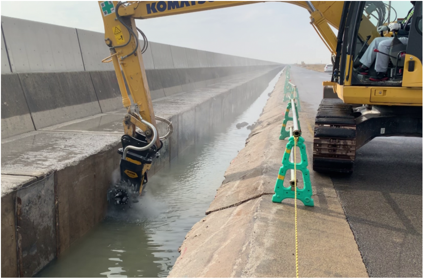
MB-R800 & Komatsu PC138 - Japan - Utility works - Concrete
