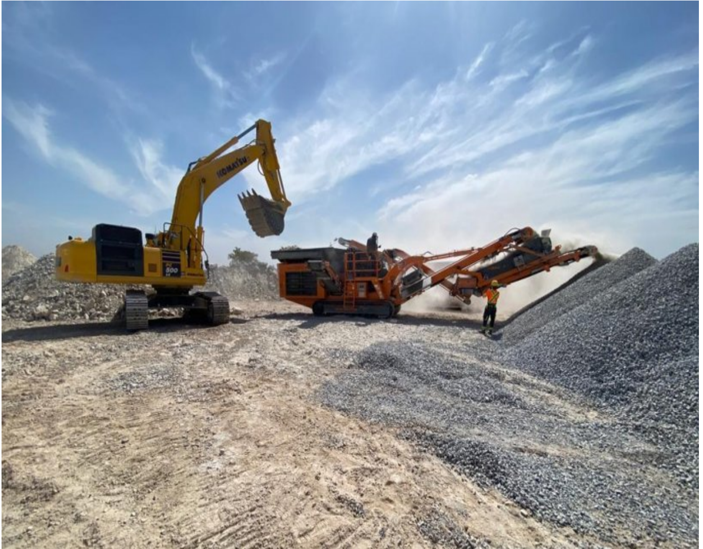
Crushing dolomite limestone with the Rockster impact crusher R1100S to 0 / 32mm. The high-quality, cubic final material is later sold for cement production.
