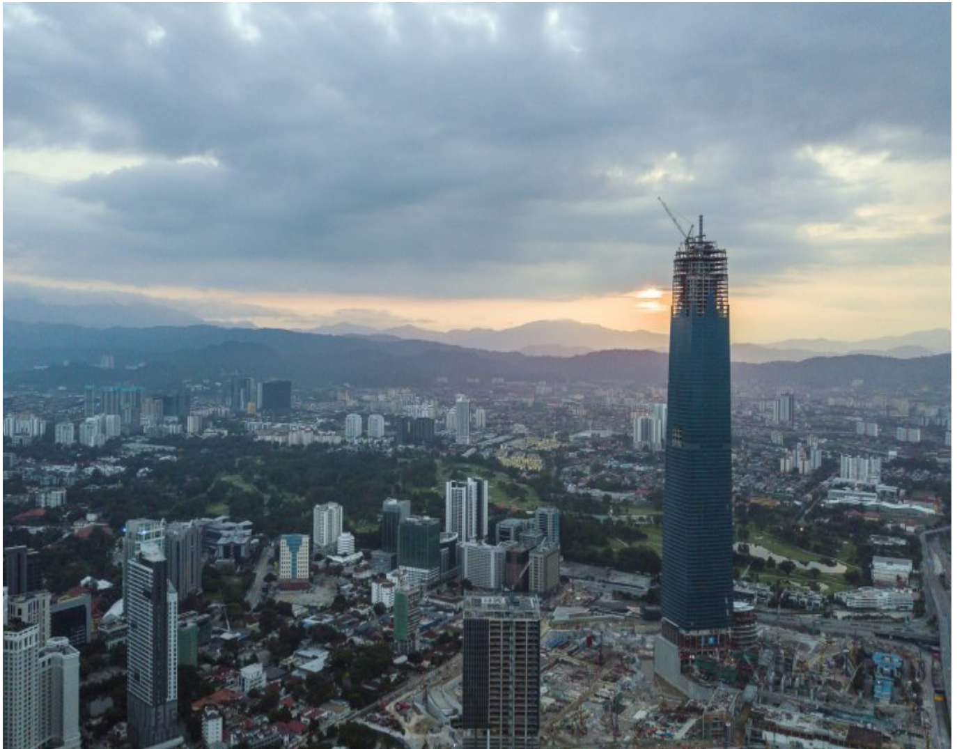
Eurotec machines keep South East Asia's tallest building on track
