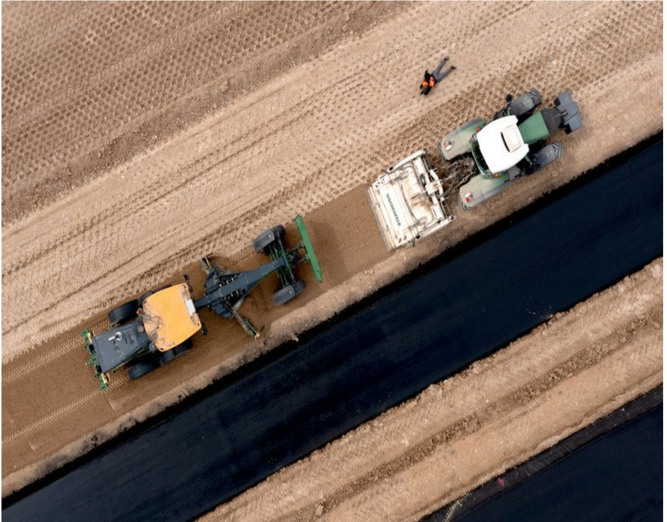
A Wirtgen Group machine train on a landfill construction project in the Kassel District of Germany
