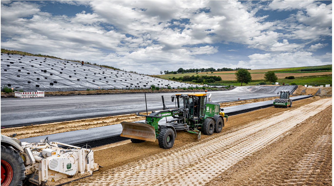
A Wirtgen Group machine train on a landfill construction project in the Kassel District of Germany
