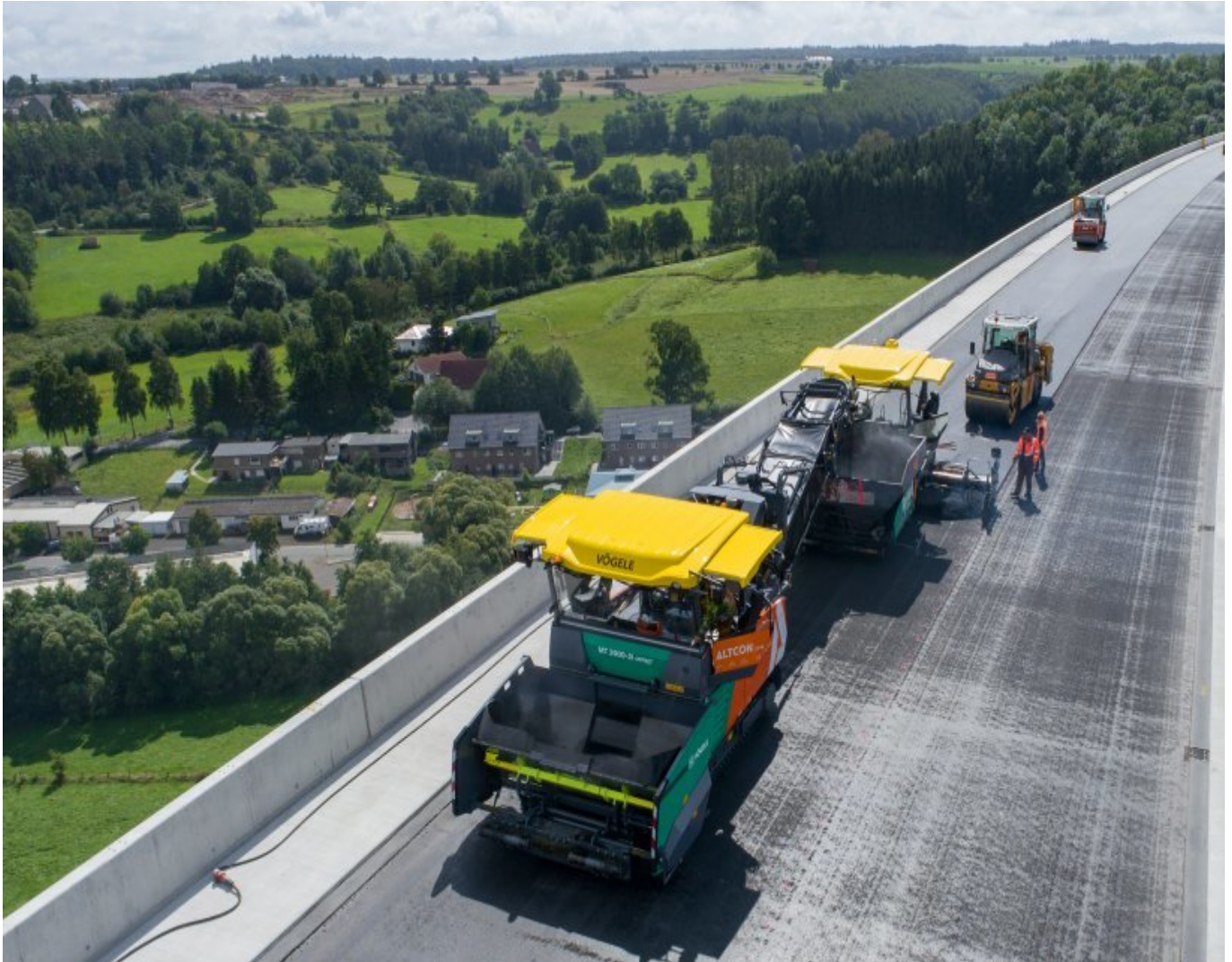
Latest-generation Vögele machines: the paving team were able to pave the surface course efficiently and to a high standard of quality using the SUPER 1800-3i road paver and MT 3000-3i Offset PowerFeeder.
