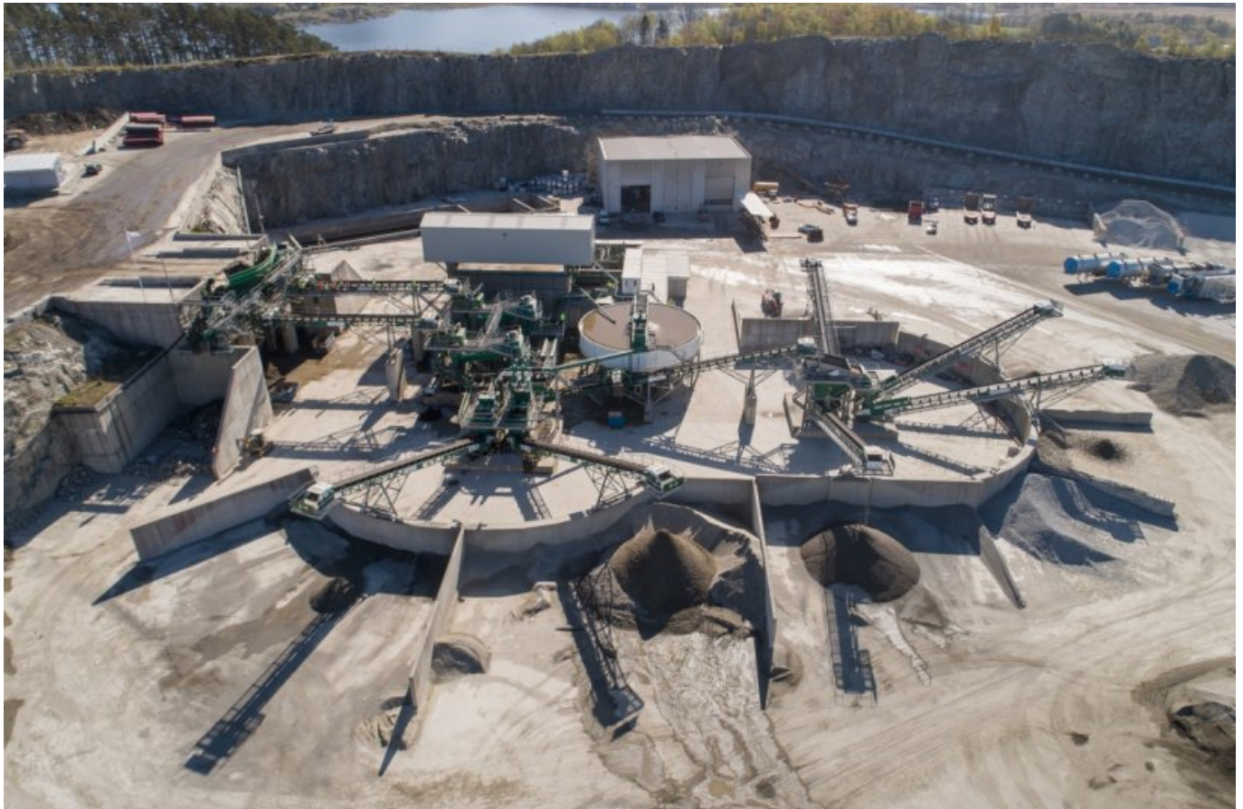
CDE - Overview of Velde Pukk Waste Recycling Facility
