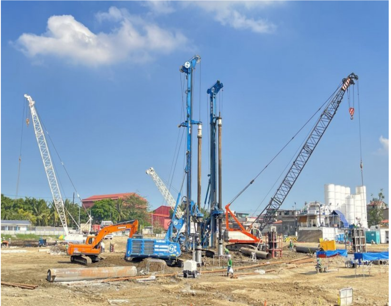
Trevi Foundations Philippines, Water Reclamation Facilities
