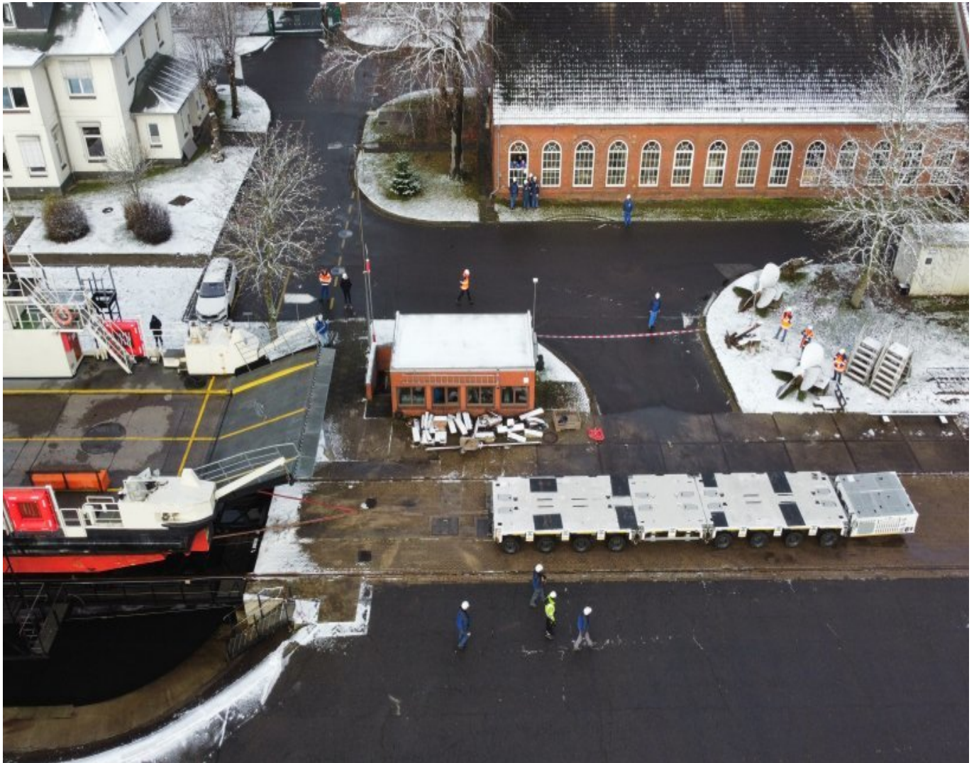
The PST/SL-E self-propelled module towing the ferry on the upper cradle ashore
