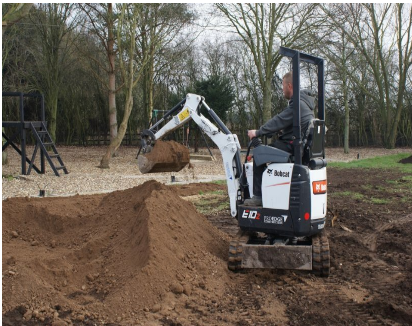
ProEdge Construction Covers East Anglia with Bobcat Fleet
