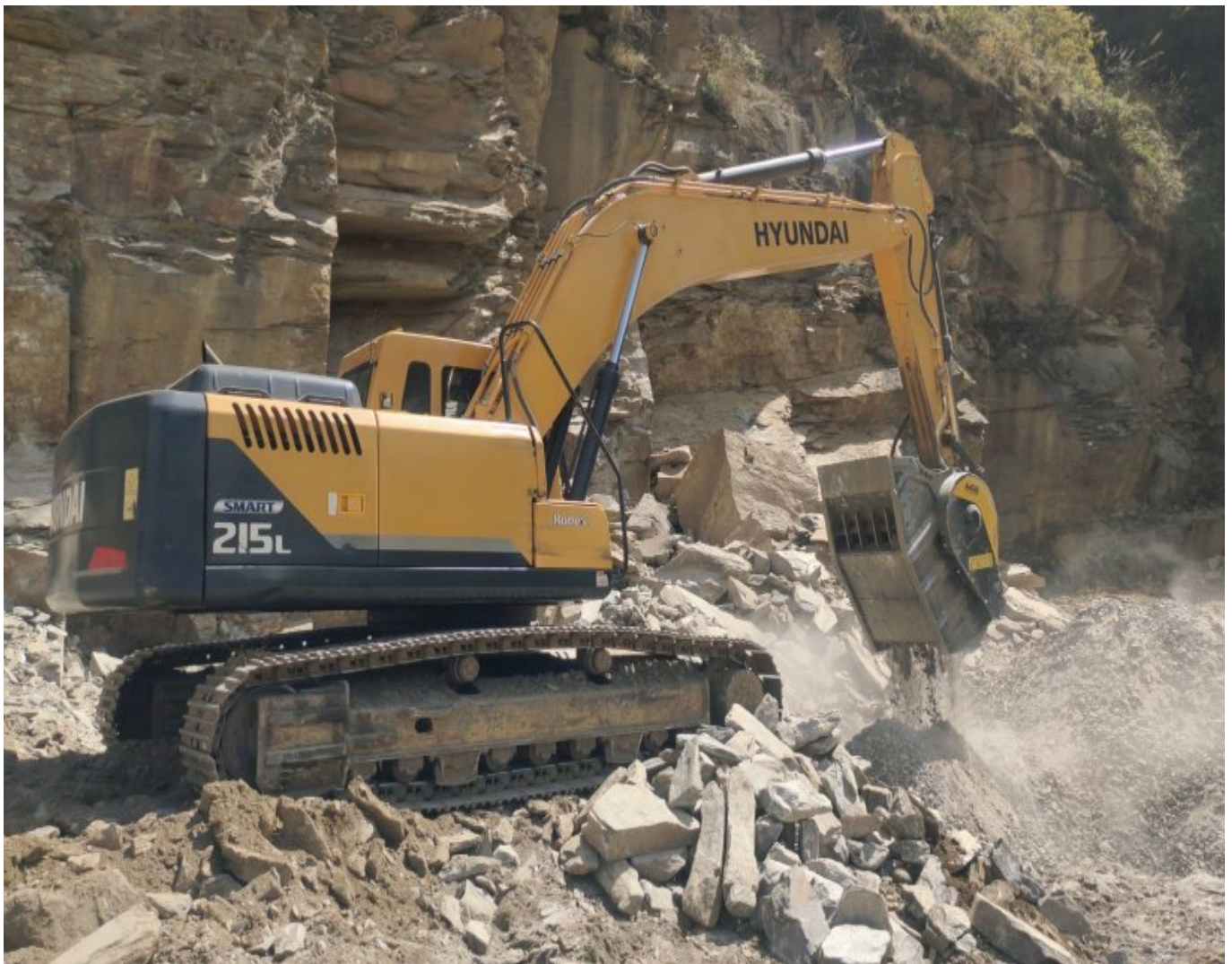
BF90.3 - Hyundai R215 - India - Road works - Hill Rock Stone
