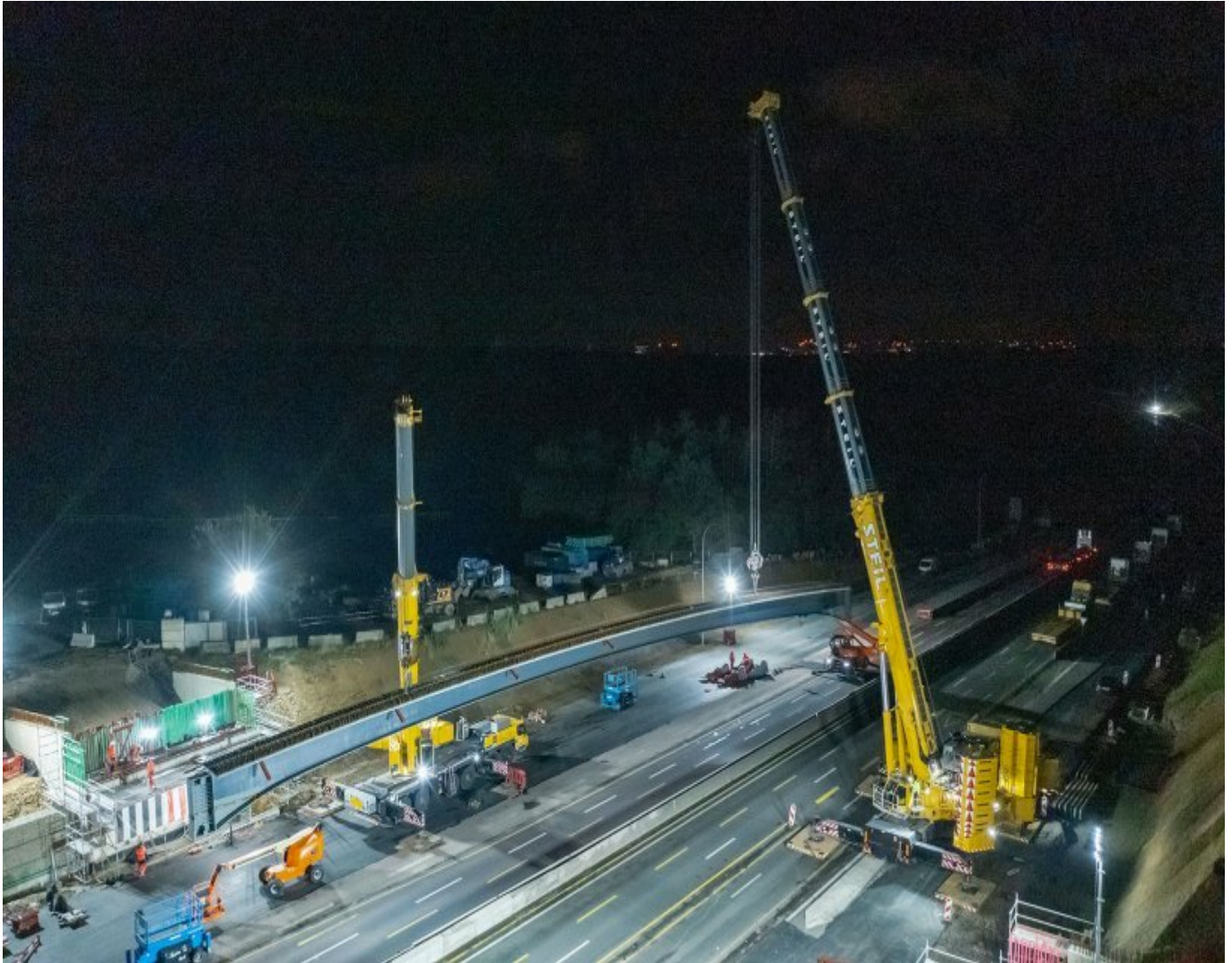
Crane duo: the Liebherr LTM-1300-6.3 and Liebherr LTM1650.8.1 lift the 92-tonne middle bridge girders on the A3 near Berchem/Luxembourg.
