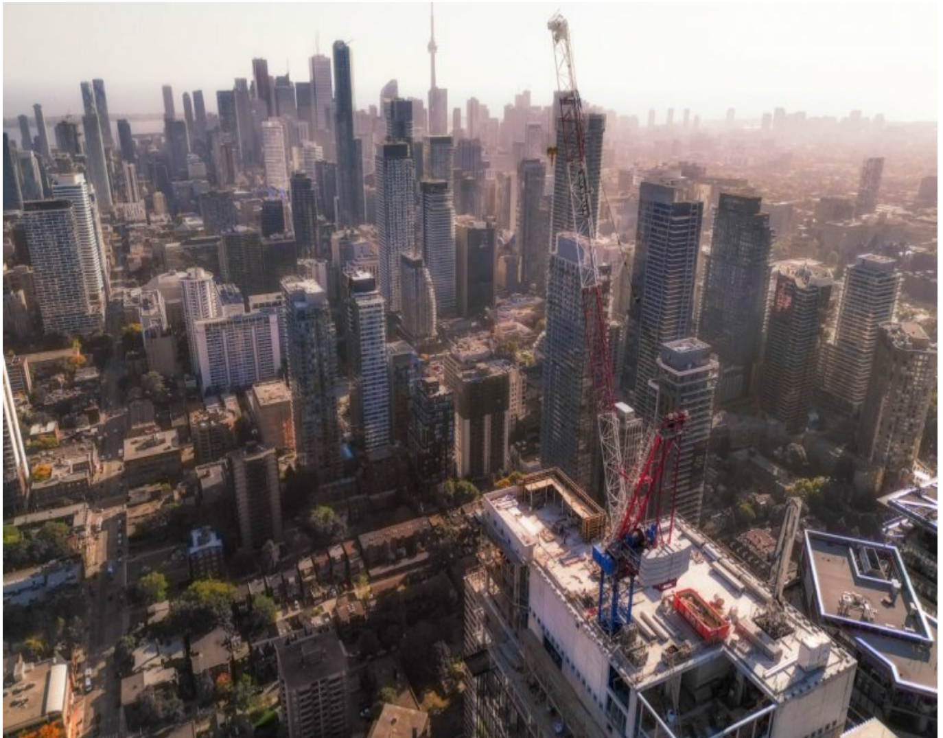
Raimondi LR273 luffing jib crane building one of Toronto's newest luxurious Condos
