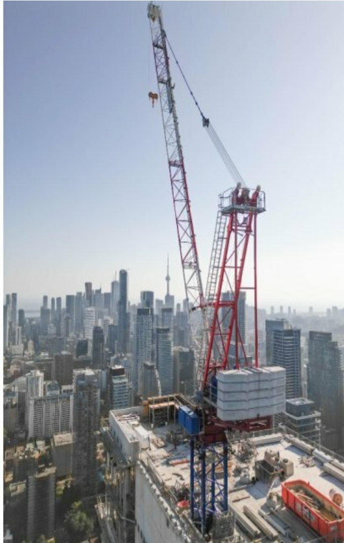
Raimondi LR273 luffing jib crane building one of Toronto's newest luxurious Condos
