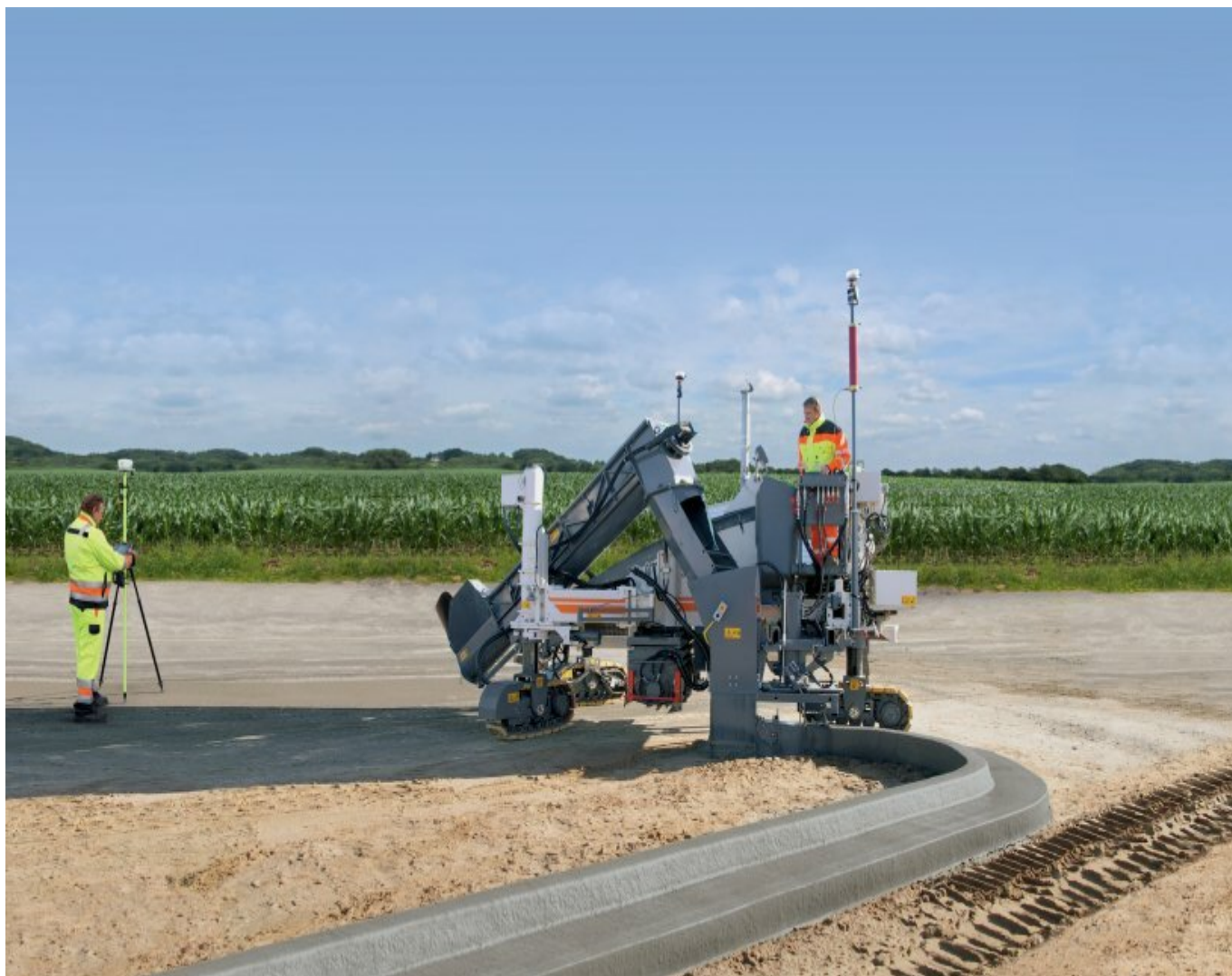
The Wirtgen AutoPilot 2.0 for stringless paving increases process efficiency and safety.
