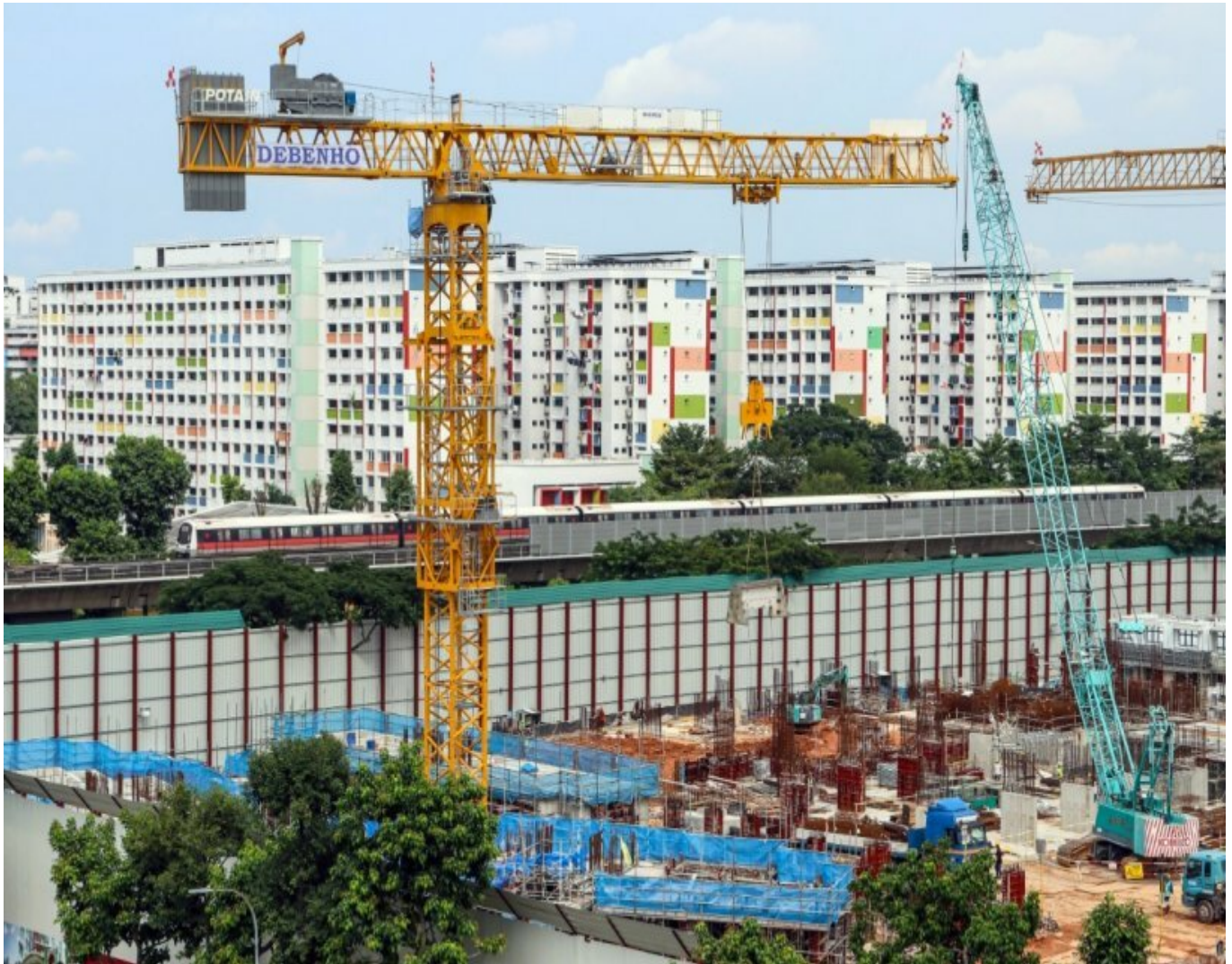
Singapore's first Potain MCT 1005 helps advance prefabricated construction
