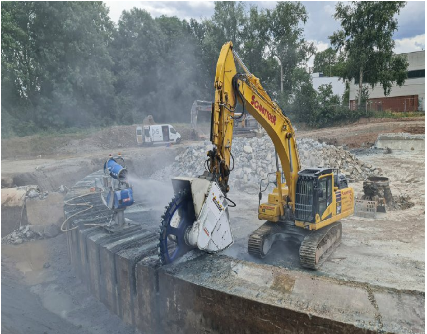
Massive concrete structures were cut up using KEMROC cutting wheels, among other things, to create space for a new residential quarter in Weingarten.
