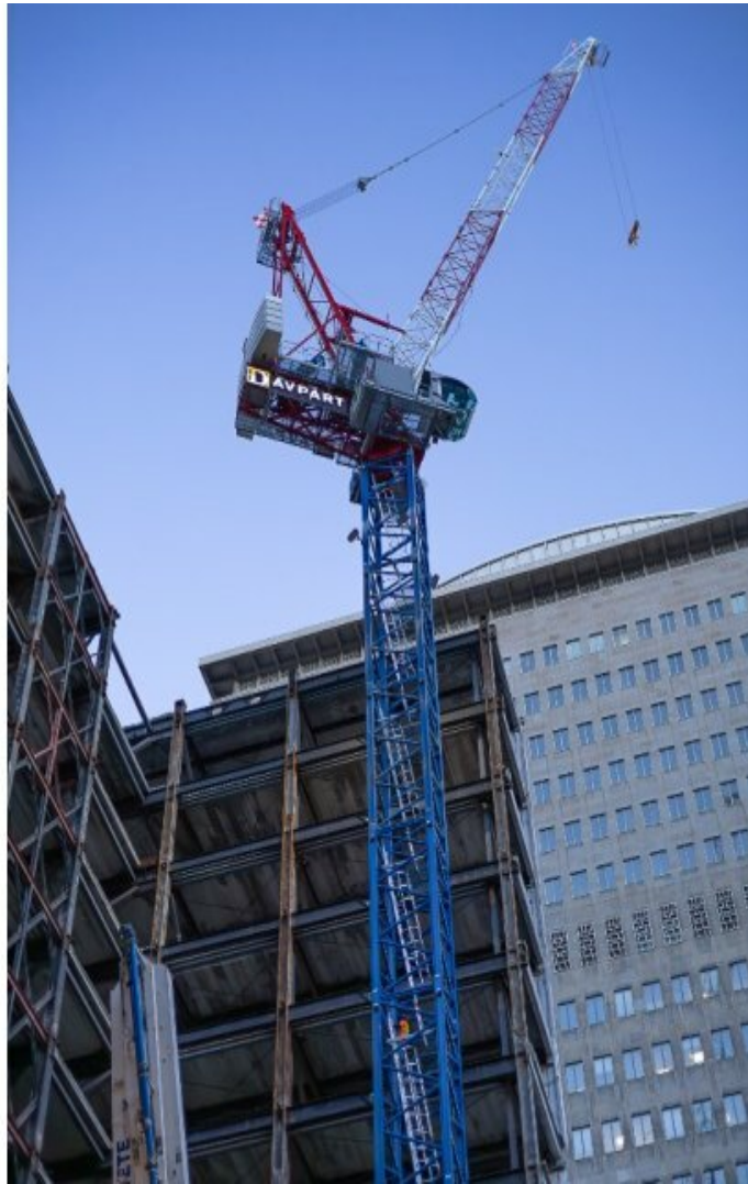
Two Raimondi LR273 luffing cranes for landmark development in Toronto
