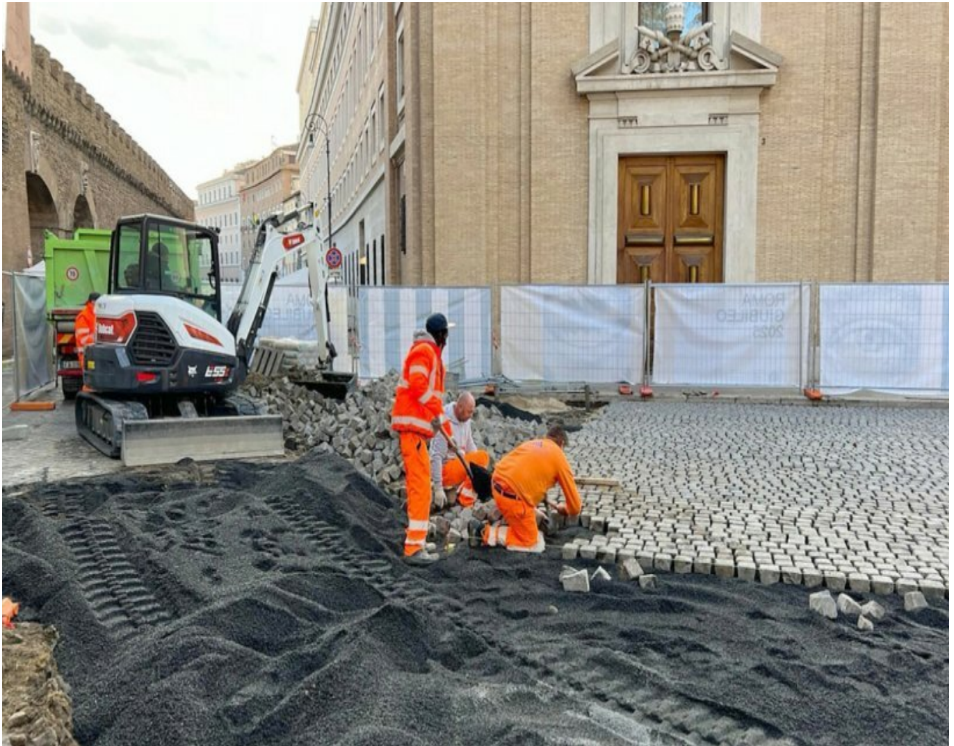
Job site - Bobcat machines at work
