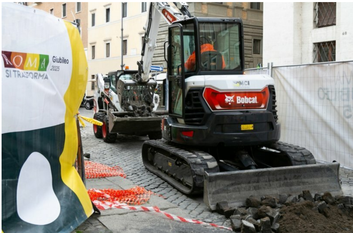
Job site - Bobcat machines at work
