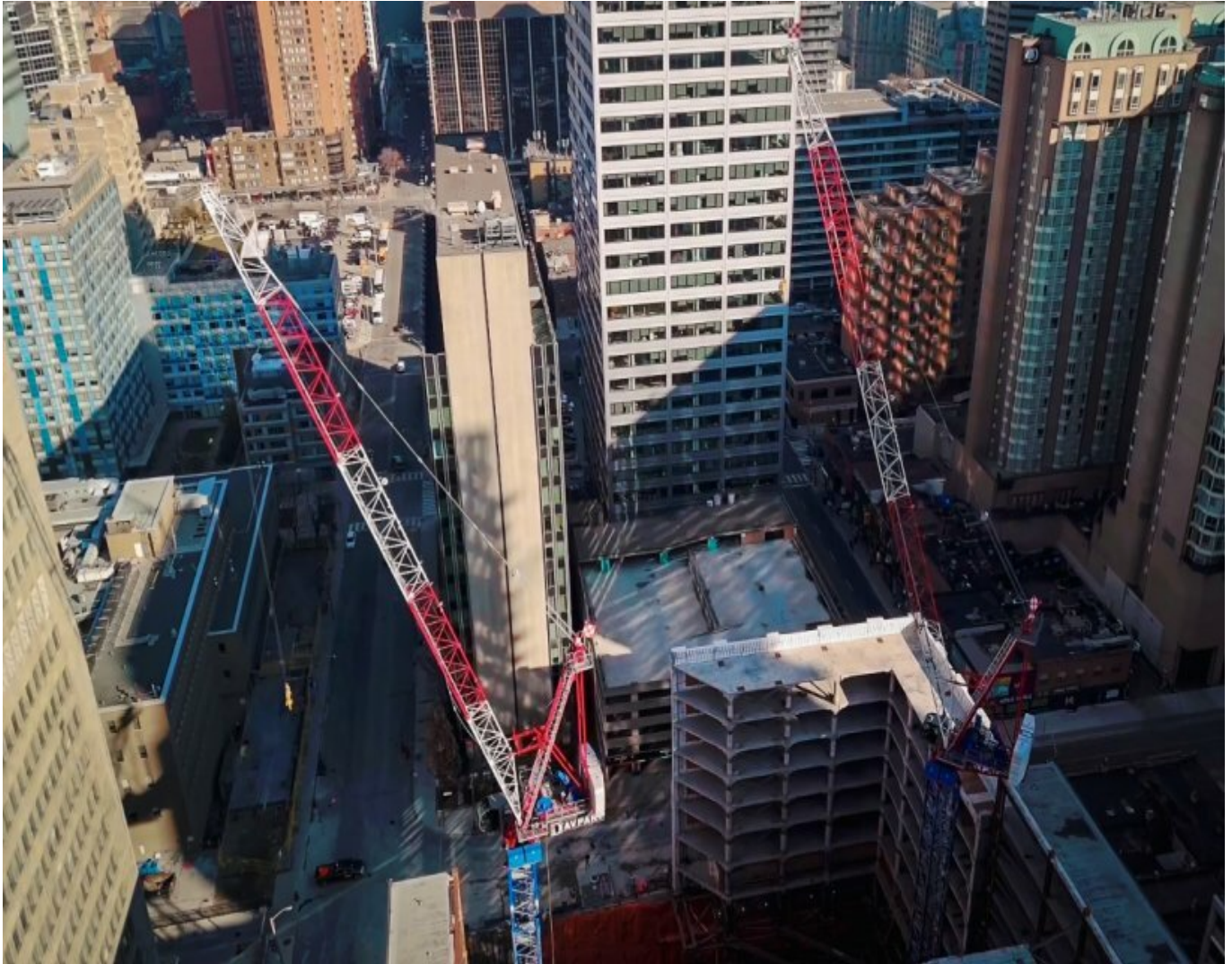
Two Raimondi LR273s for North America's largest heritage redevelopment
