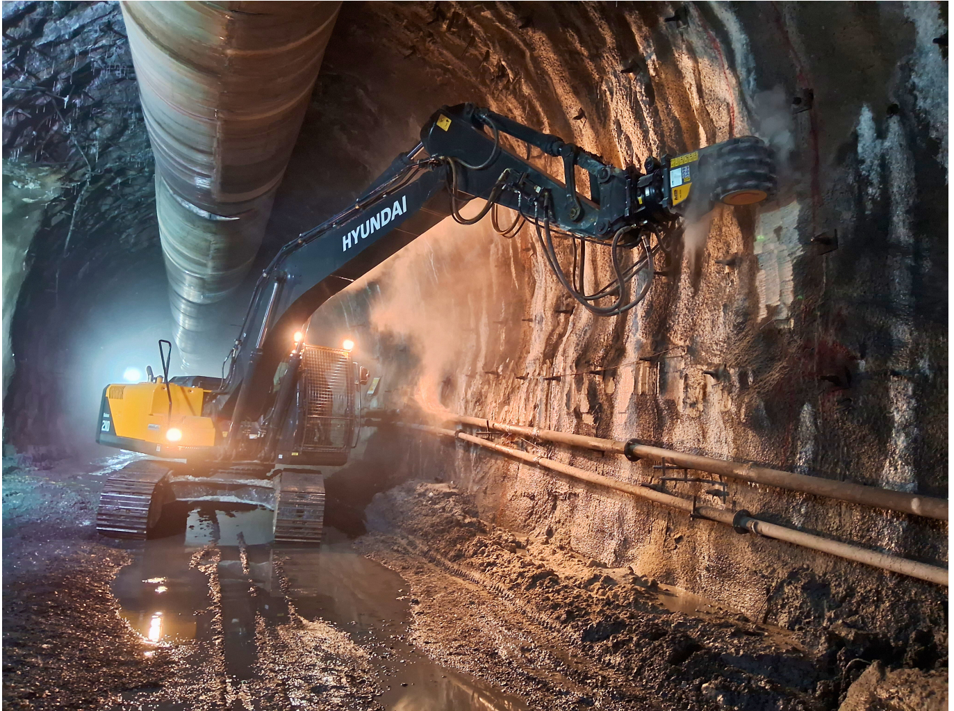
MB-R500 - Hyundai R210 Smart - India - Railway project - Concrete
