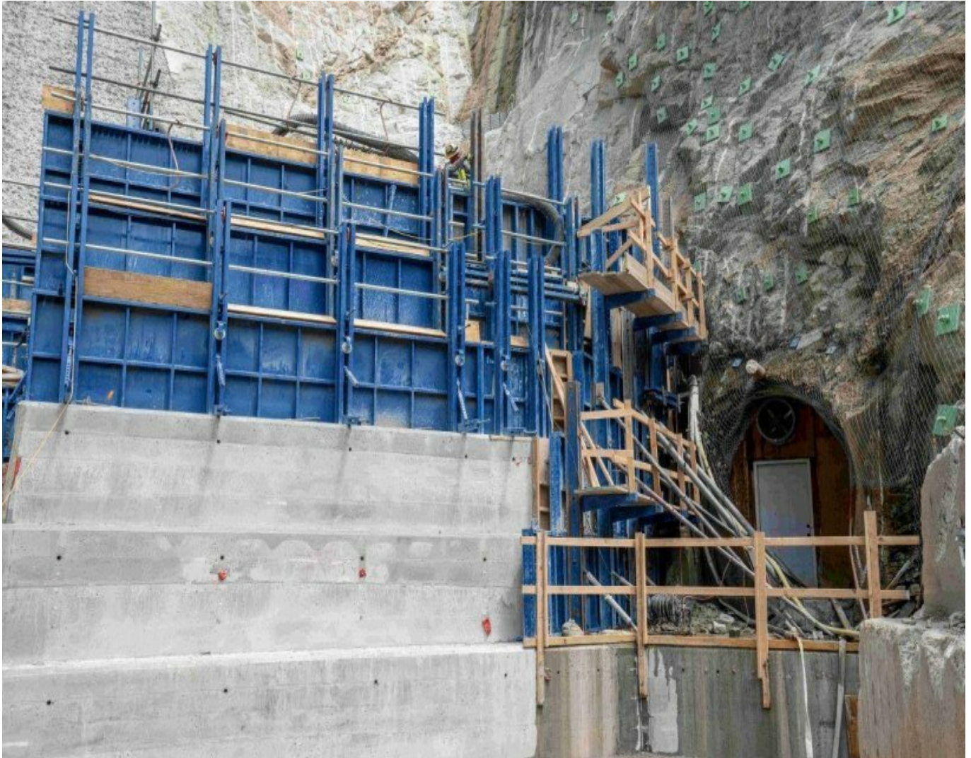
Doka custom formwork for roller compacted concrete.
