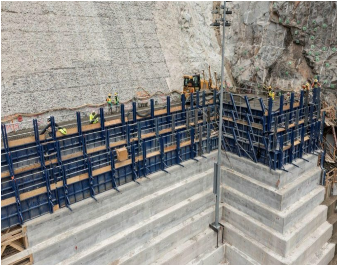
New dam steps are formed using Doka's custom girder system.
