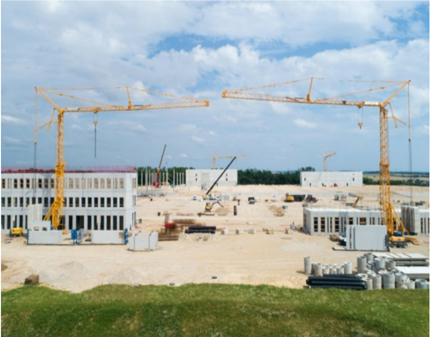
SOFIALEX completes fast-track build with Potain Igo T 130 cranes
