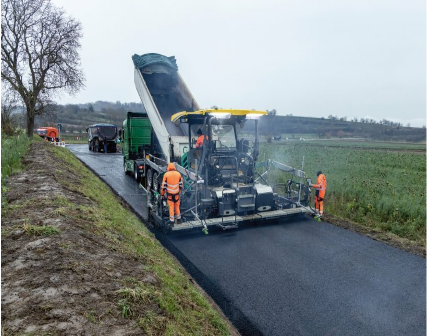
Construction contractor Johann Joos Tief- und Straßenbau GmbH rehabilitated a 1.3 km section of the L 106 country road between Wagenstadt and Bleichheim with the new SUPER 1800-5i paver from Vögele.
