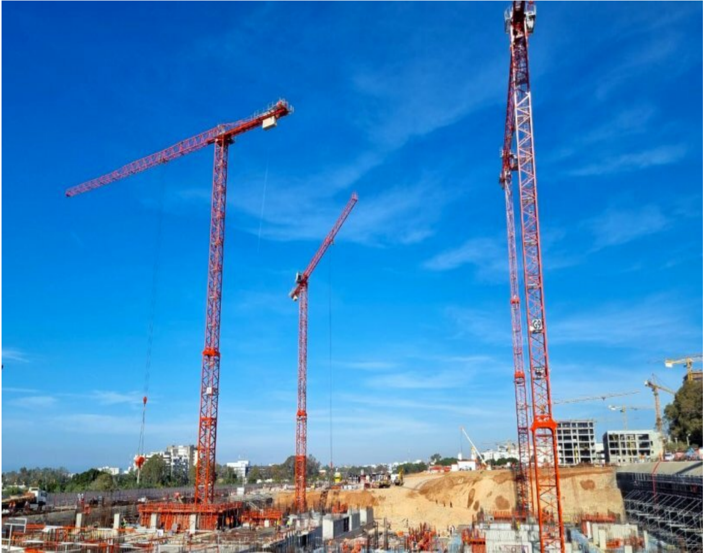
Manitowoc and PROMAT building North Africa's future together
