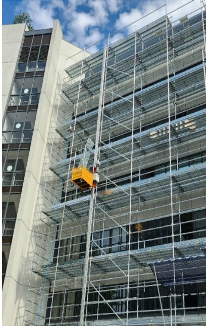
Alimak STS 300 - Scaffold Transportation System in action
