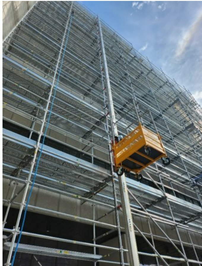
Alimak STS 300 - Scaffold Transportation System in action
