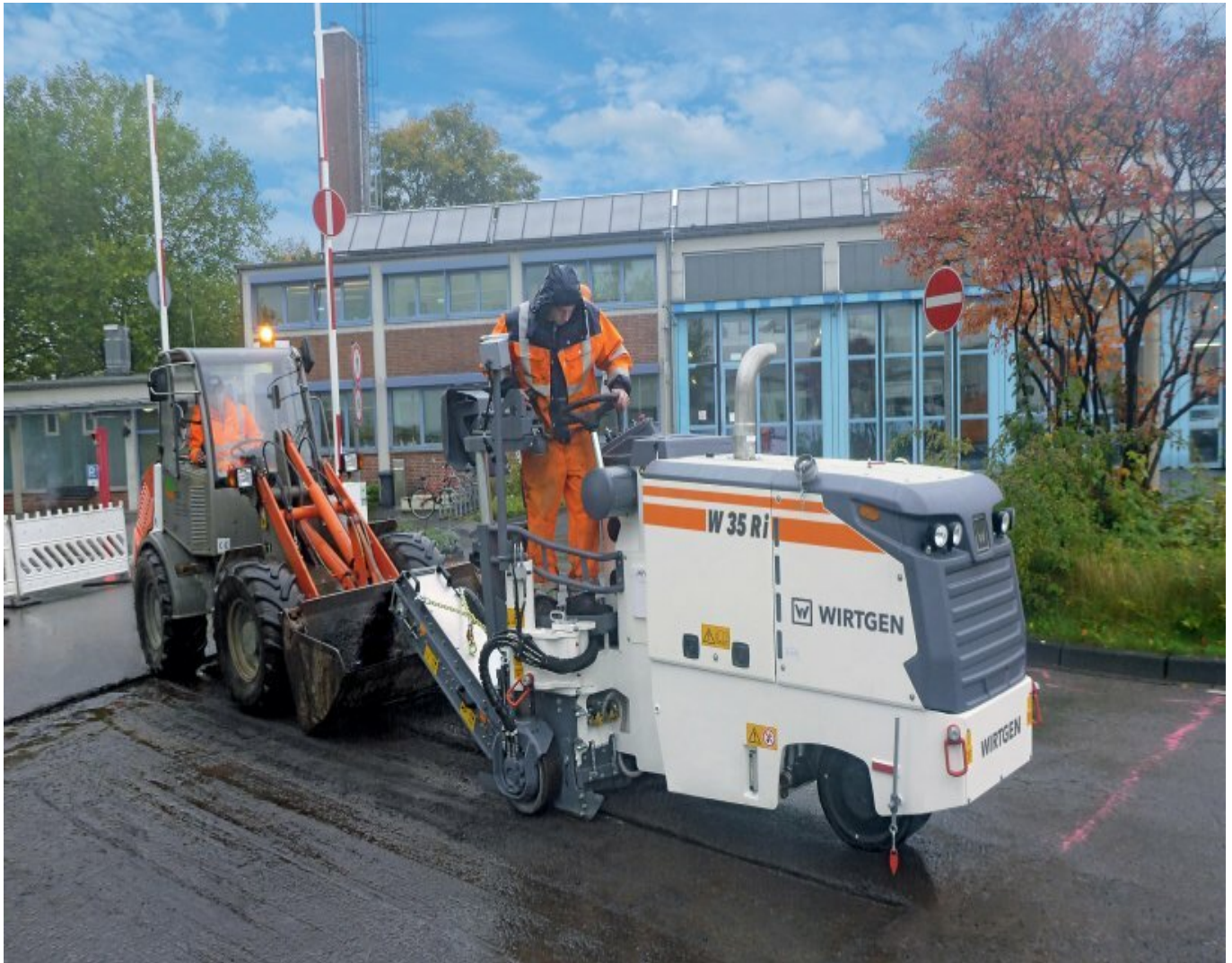
The Wirtgen small milling machine W 35 Ri rapidly mills off the surface layer or even several layers at a time.
