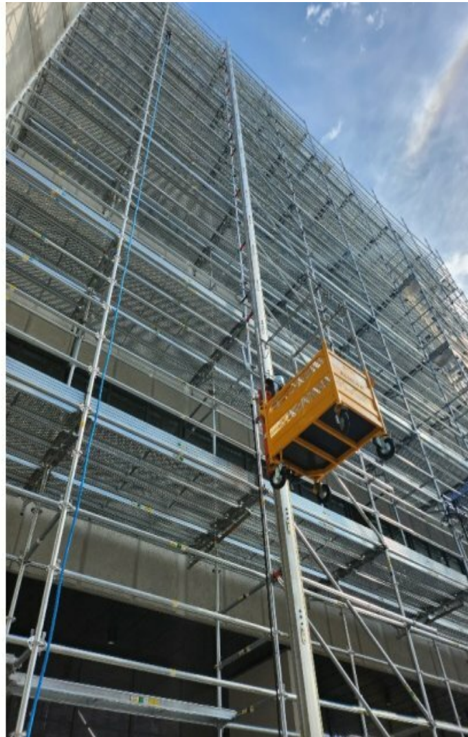
Alimak STS 300 - Scaffold Transportation System in action
