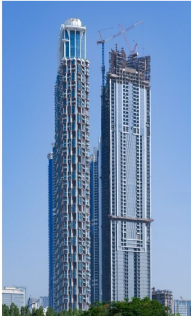
Raimondi LR213 elevates Dubai's skyline to new heights with highest climbed crane in the region
