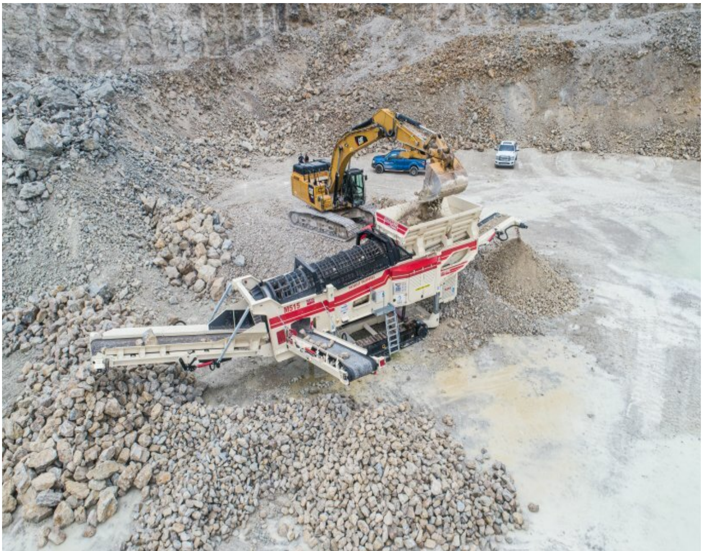
The M515 in action, processing rip rap, destined for use in a shoreline restoration project.
