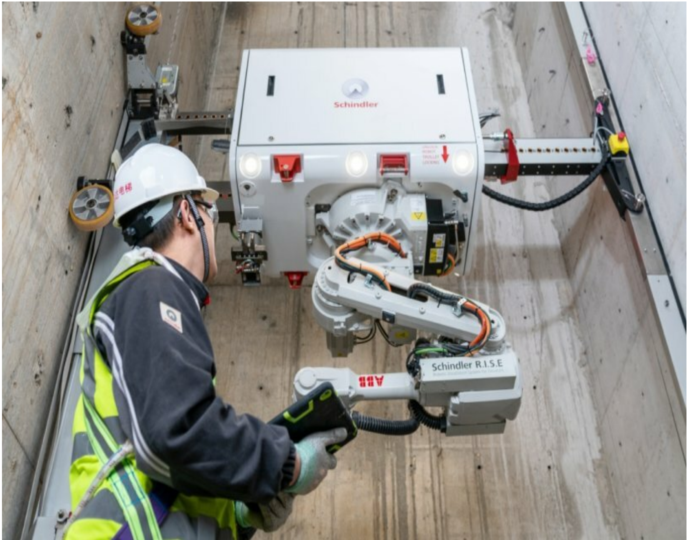
Advanced Schindler R.I.S.E construction robot in Singapore to support Shaw Tower redevelopment
