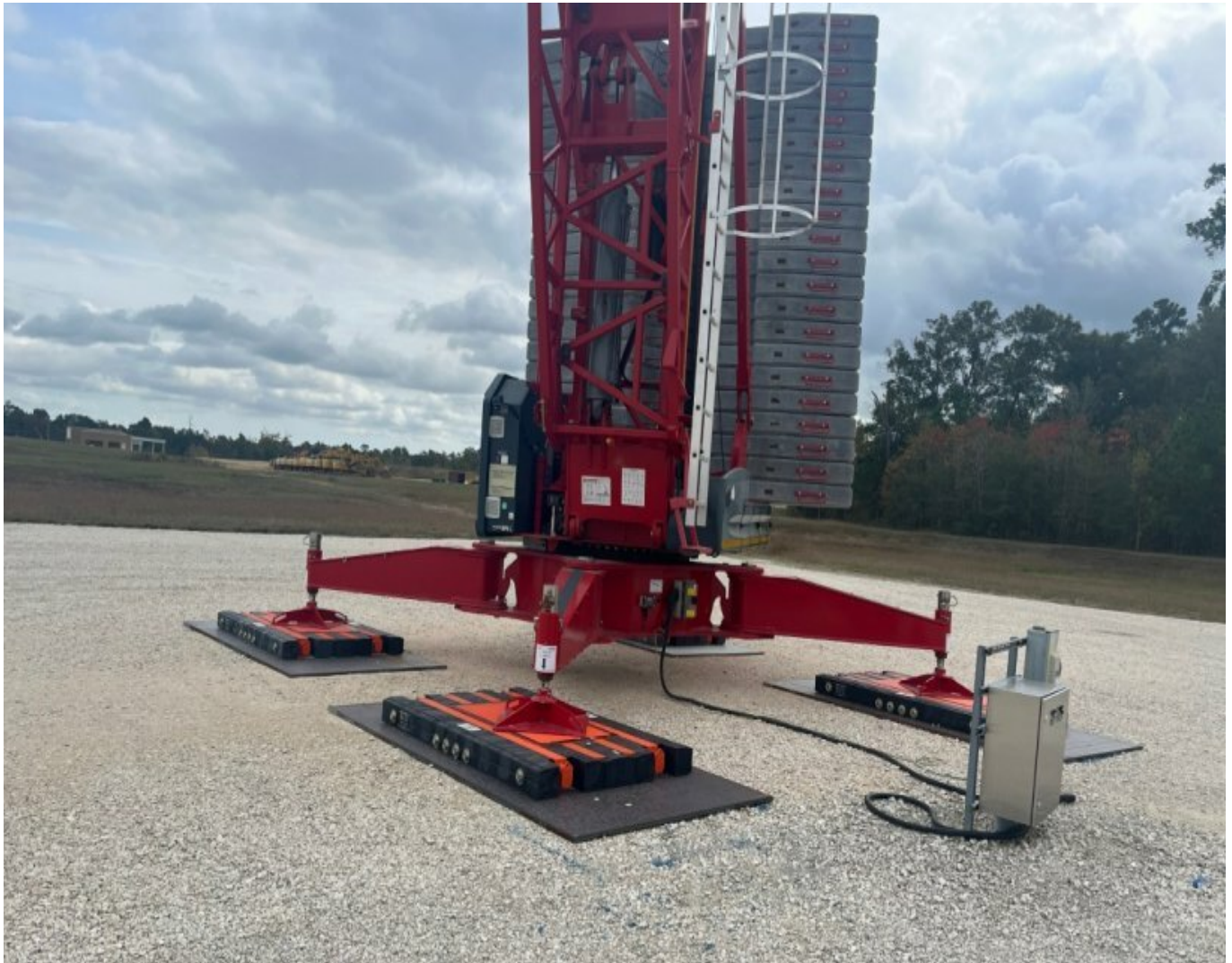
IUOE Sets Up New Self-Erecting Tower Crane at Training Center on DICA EcoMax Crane Pads
