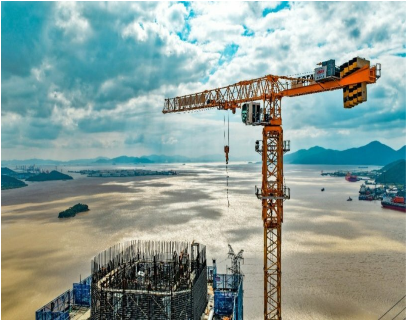
Potain MCT 385 cranes support construction of the world's longest-span road-rail bridge
