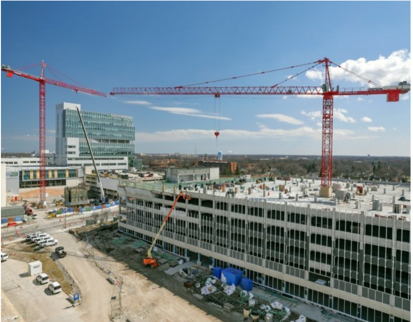
Two scopes, two cranes, one campus: Potain tower cranes support major hospital-campus build in Milwaukee
