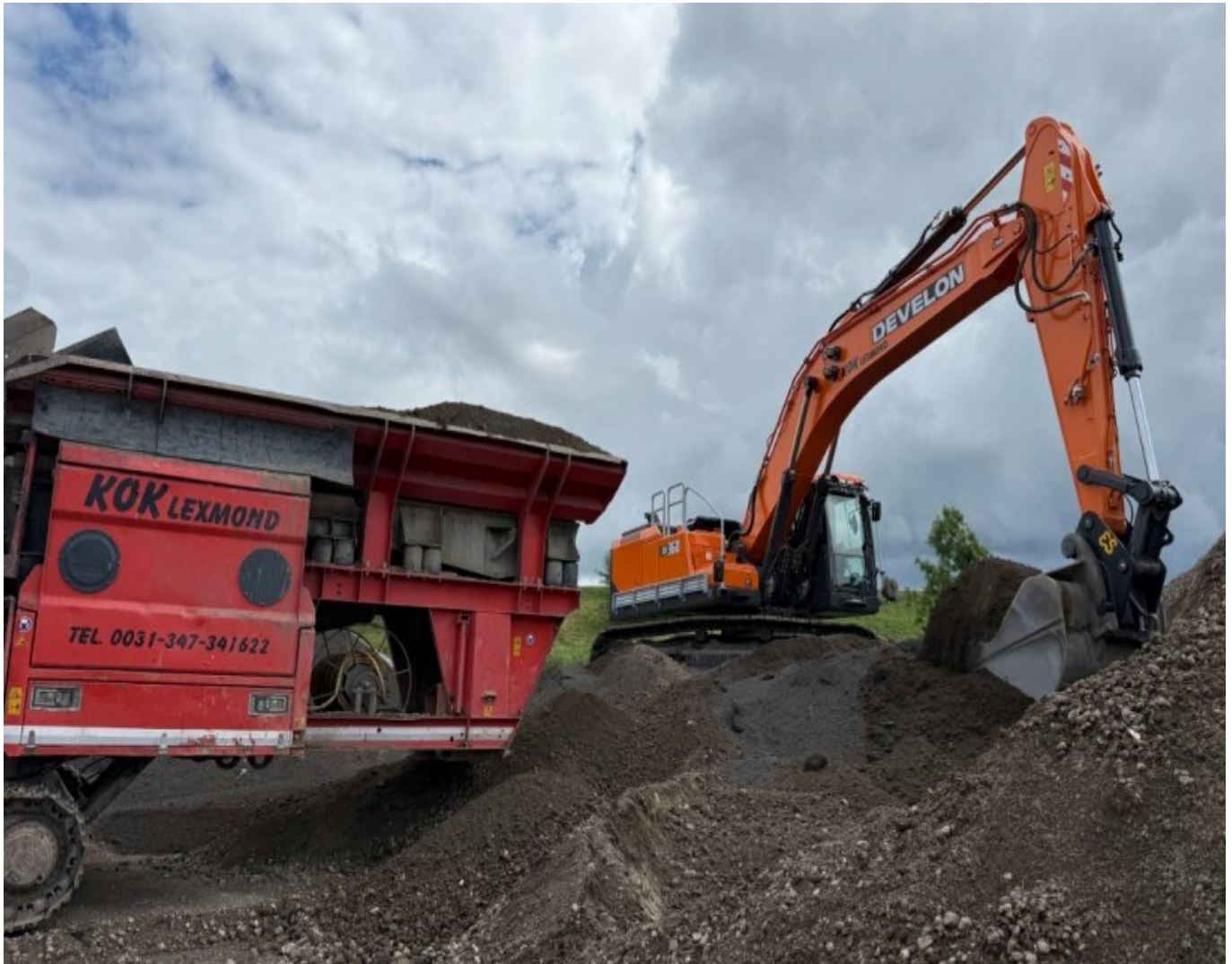
Develon DX360LC-9 Smart Crawler Excavator
