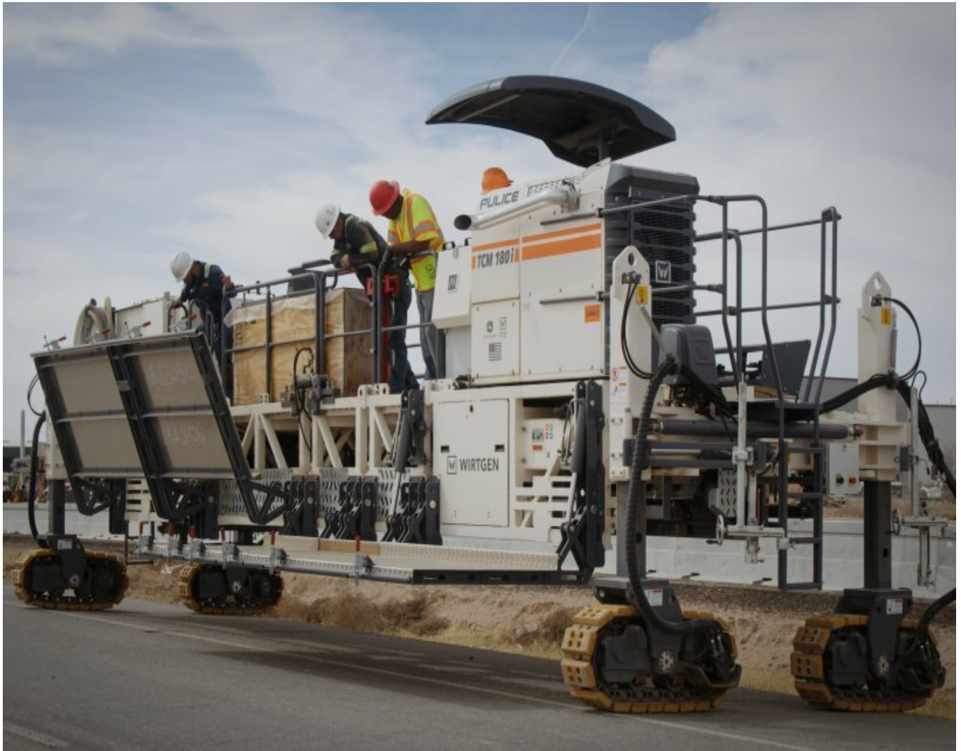
The self-propelled texture curing machine TCM 180i produces the desired surface textures on the freshly paved concrete pavement.
