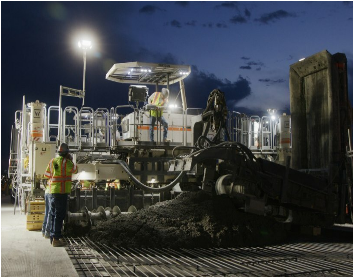
Wirtgen WPS 102i: The 2-track placer/spreader places and spreads concrete at widths of 4 to 12 m and a thickness of 500 mm in front of the paver.
