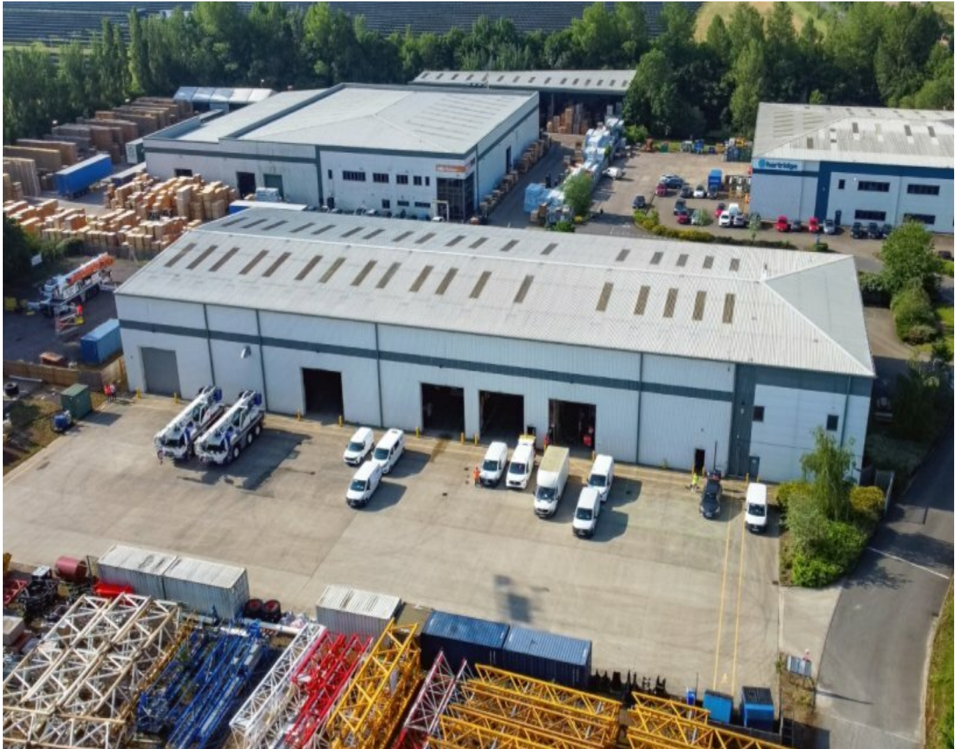
The MGX facility in Buckingham, UK
