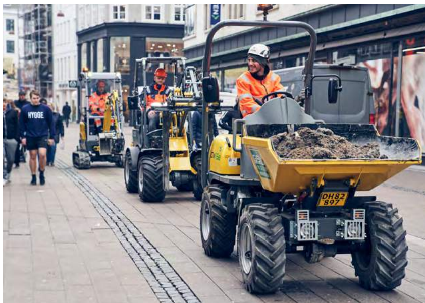
Electric and battery machines in action, Copenhagen
