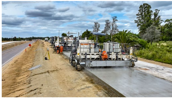
The texture curing machine TCM 180 followed on directly behind the SP 64 and produced the desired texture for the concrete road surface. In addition, a dispersion was simultaneously applied to prevent premature drying of the surface and edges. Image source: Wirtgen Group
