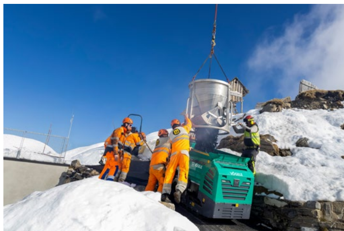
The helicopter transferred the mix directly into the material hopper of the Vögele paver. Image source: Wirtgen Group
