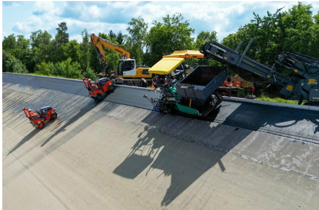
Wirtgen Group machines impress as a universal solution – here with a particular focus on the two Hamm rollers that precisely compacted the steeply sloping surface. Image source: Wirtgen Group
