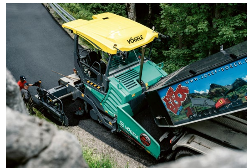
The Vögele road paver and the Hamm rollers had to be steered with absolute precision through the narrow serpentine to achieve the best possible result. Image source: Wirtgen Group
