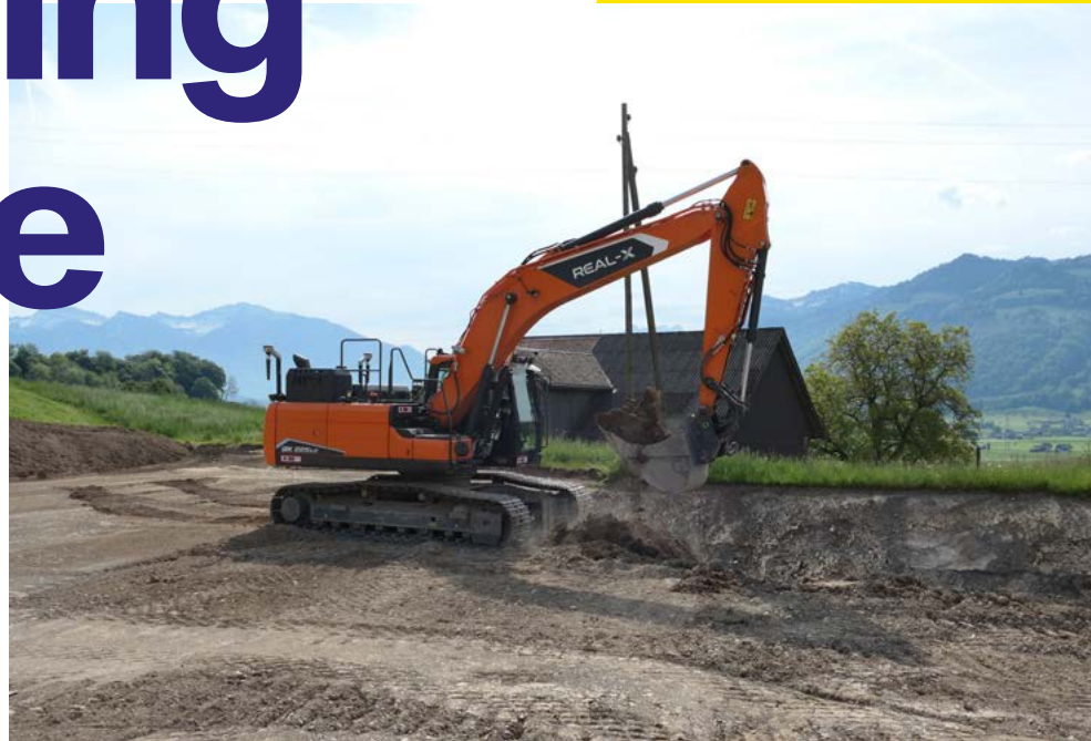
A magnificent backdrop: the autonomous DEVELON Real-X DX225LC crawler excavator in action at the former KIBAG quarry in Tuggen, Switzerland. Image source: DEVELON
